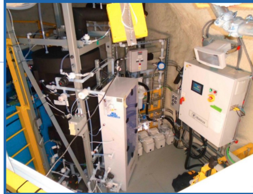
Scintillator, TeA, TeBD purification plants underground
