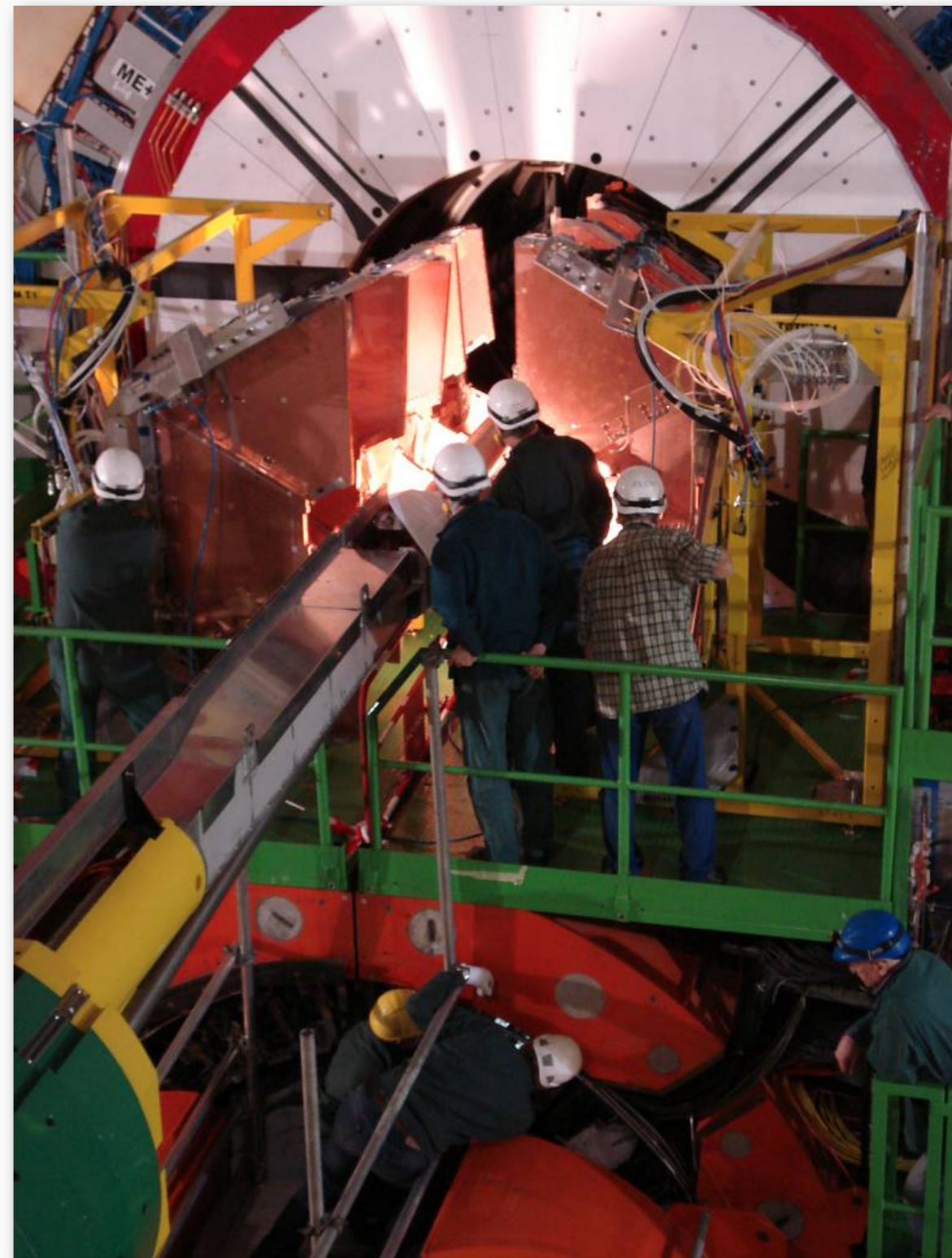
Installation of 2'nd T1 telescope
