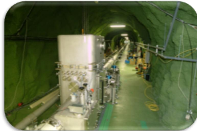
The world's first demonstration of cryogenic system for interferometer
