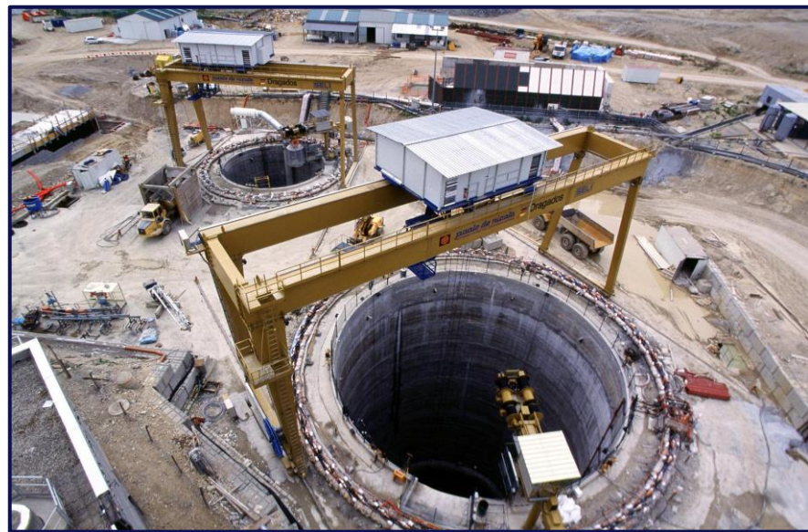
Ground Freezing used on Previous CERN Shafts
