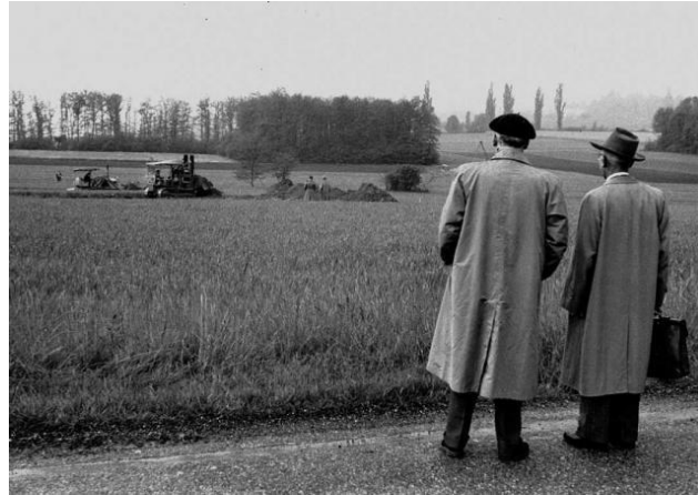
Start of Civil Engineering March 1954
