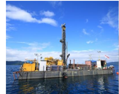
Drilling works on the lake
