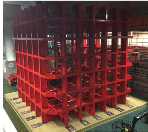
Beam structure assembly completed
