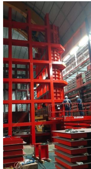
Tertiary membrane panels installation
