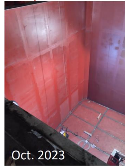
Tertiary membrane panels welding
