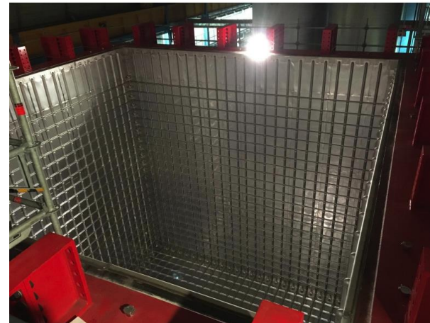
Primary membrane welding
