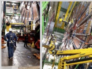
4: Hoist with crane
