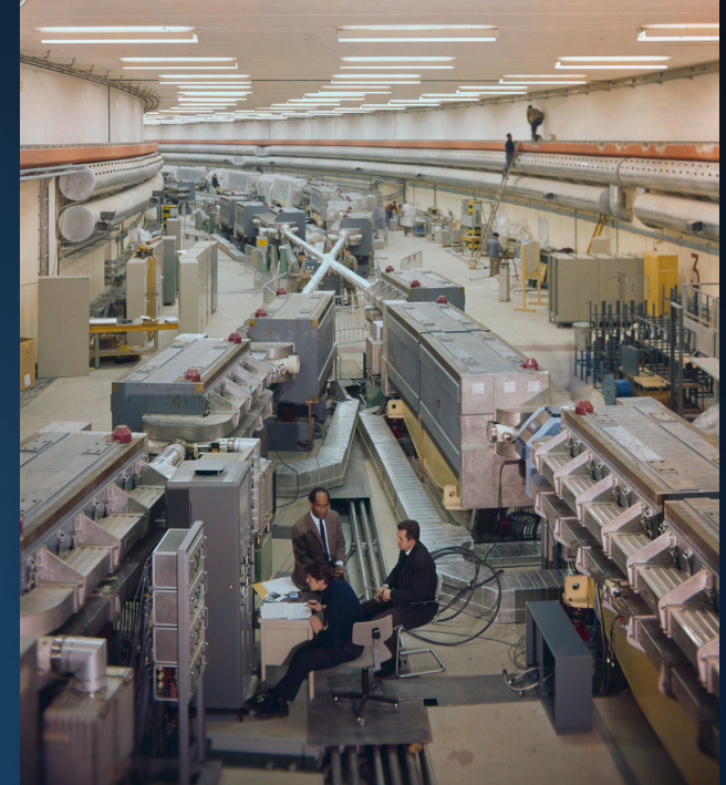
Intersecting Storage Ring
