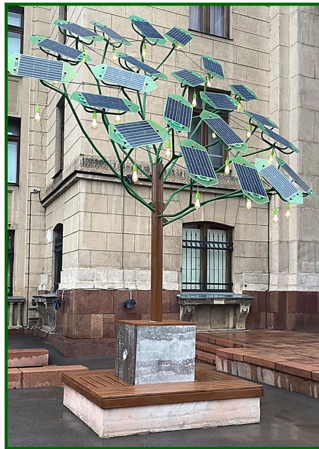
Solar Tree with a power of 0.5 kW
