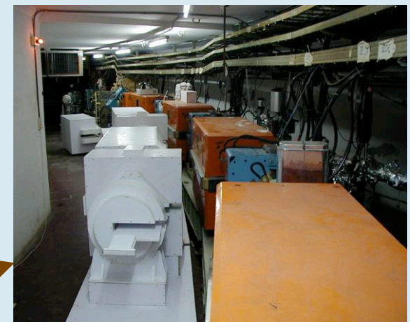
Two rings tunnel
