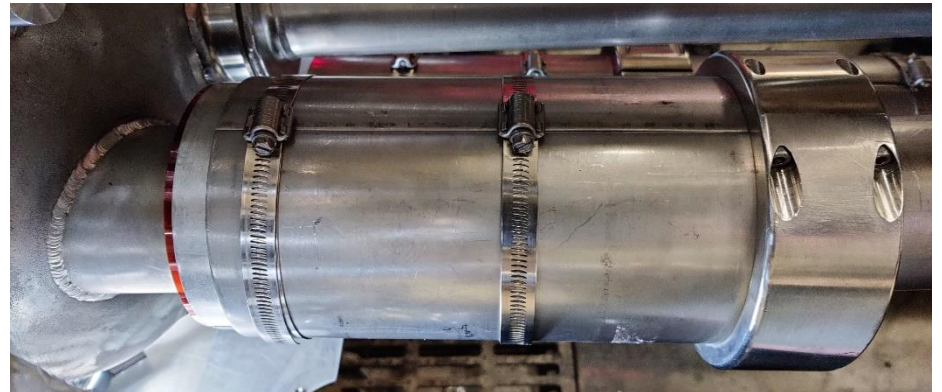
Bellows is surrounded by 3 layers kapton, then aluminium + stainless steel guide shells
