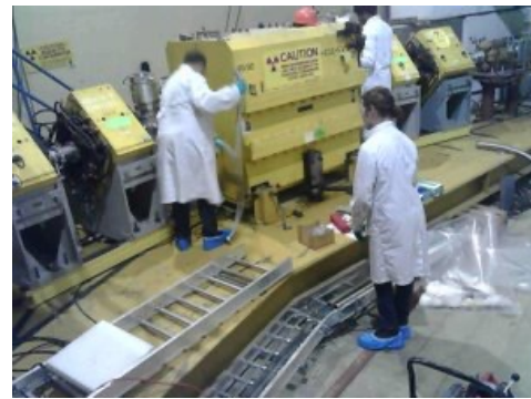
BL4N vault installation
