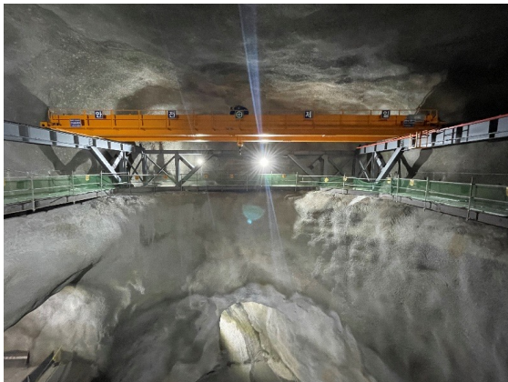
LSC Hall 10-ton crane • Completion June 2023
