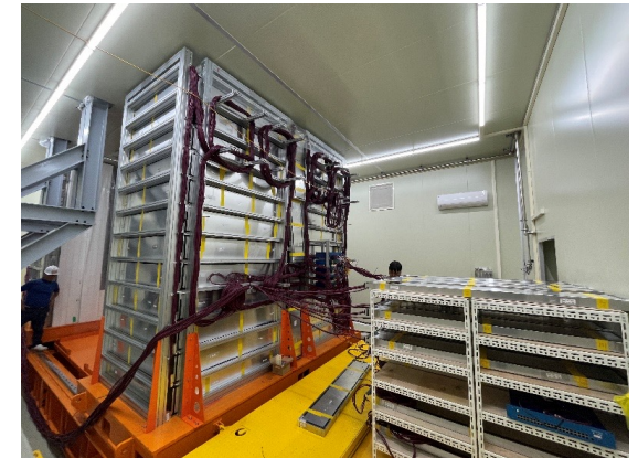
AMoRE-II • Shield structure done • Late 2024, commissioning
