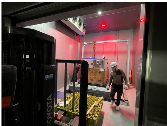
COSINE-100U • -30°C low-temp. room • Moving Y2L detector to the room • Early 2024, commissioning
