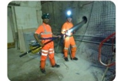
Bore hole detector installation
