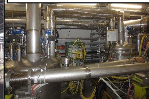
Flexible line between fixed box and moveable table
