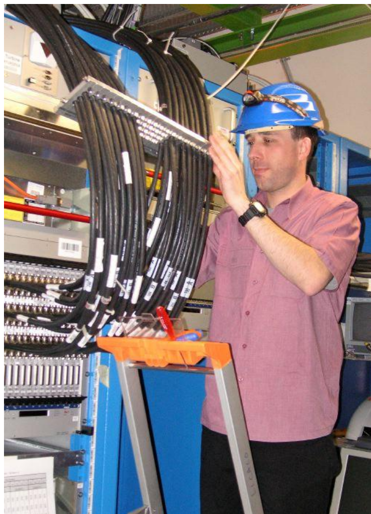
Cabling of calorimeter trigger
