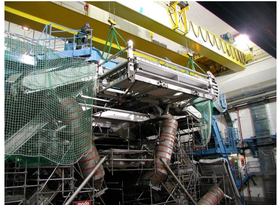
Installation of barrel muon station
