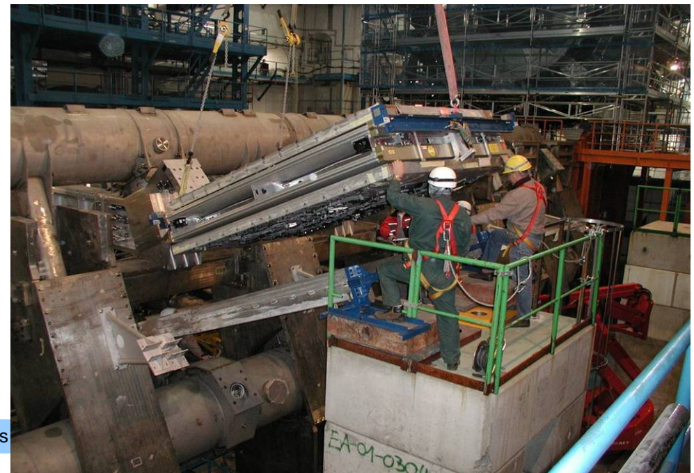
Installation of barrel muon station
