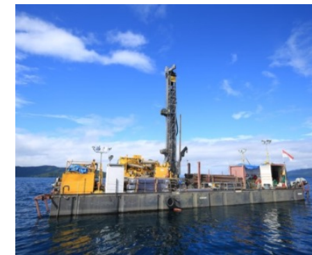
Drilling works on the lake
