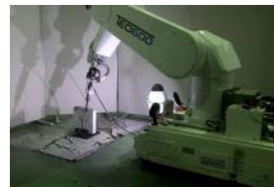
Concrete breaking by Chiselling
