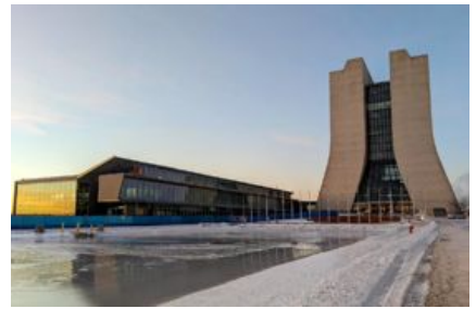
New building at Fermilab for ND-LAr construction
