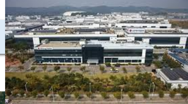
LG Energy solution (Battery company)
