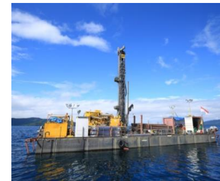
Drilling works on the lake
