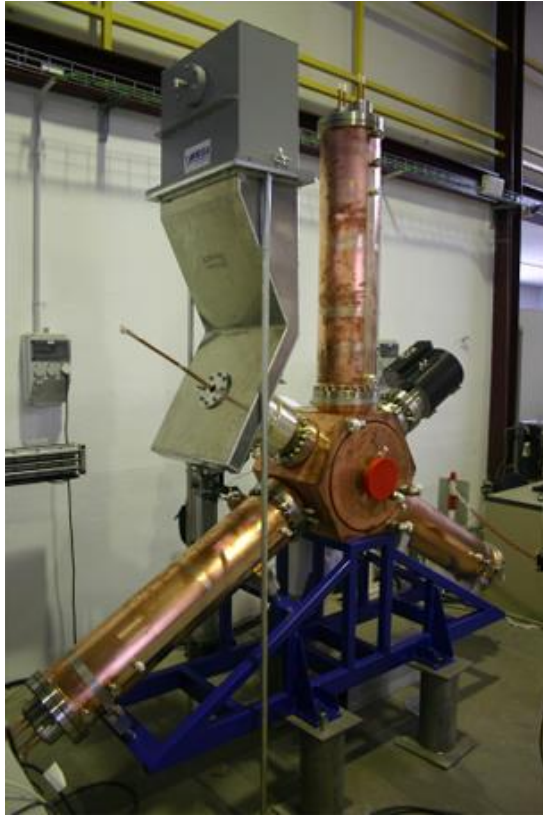
Main RF cavity (DAMPY) 600 kV max - 500 MHz
