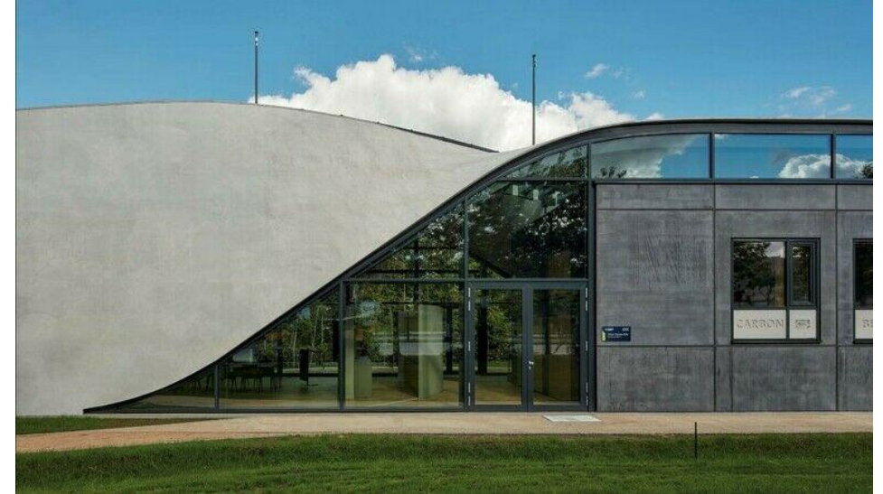
Example: Cube in Dresden - the world's first building made of carbon concrete (from: www.bba-online.de/news/cube-neues-bauen-mit-carbonbeton/#slider-intro-1 )
