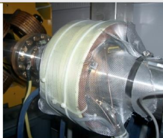
WALL CURRENT & DCCT MONITOR
