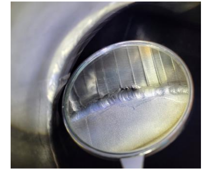
Mirror inspection. Undercut in the weld of a heat exchanger
