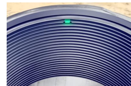
Trough PT in leaking bellow, LHC TDIS collimator
