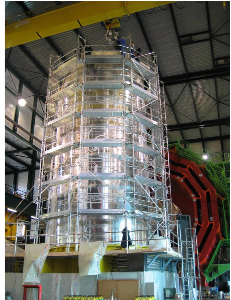
Example: CMS Solenoid thermal shield
