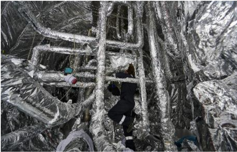
MLI (Al coated Mylar) HL – LHC's cold box
