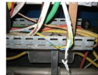
Representative examples of installed cables subjected to different total absorbed dose. CARE Project. Courtesy of J. Gascón [15]
