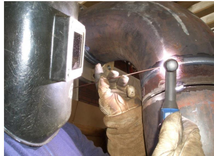
TIG Welding of Pressure Vessel
