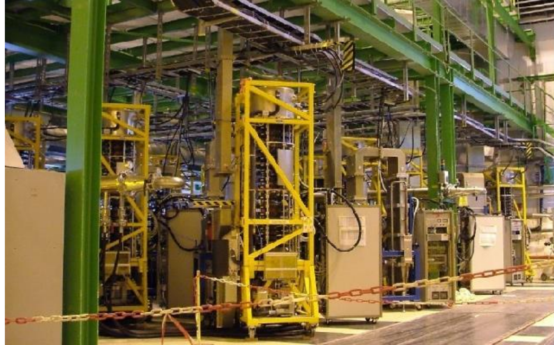
CERN LHC Power plant 16 x 330kW continuous wave @ 400MHz Based on klystron In operation since 2005 (20 years ago)
