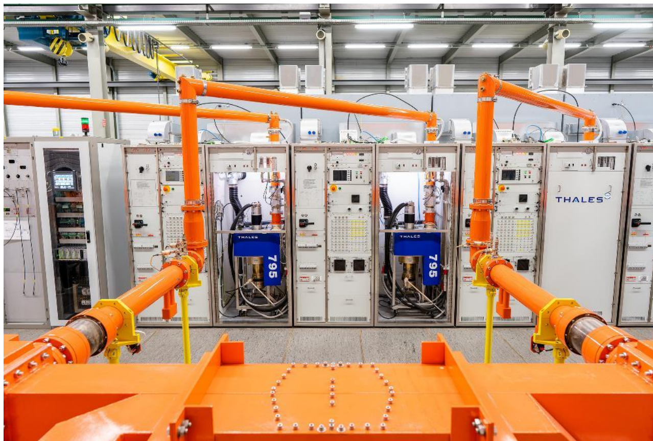
CERN SPS, TH 795 IOT, Trolley (single amplifier), and transmitter (combination of amplifiers) Two transmitters of four tubes delivering 2 x 240 kW @ 801 MHz, into operation since 2014
