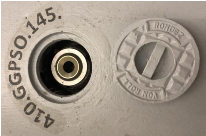
GGPSO, LHC underground geodetic network
