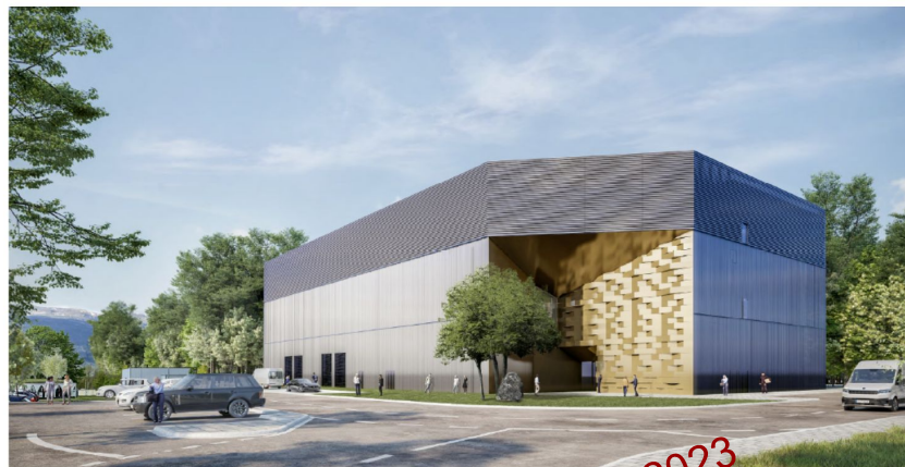
An artist's impression of the CERN Data Centre in Prévessin. The facility will consist of three floors, to be progressively filled with computing equipment over the first ten years of operation. (Credit: + IMGs - Rocco Valentines)
