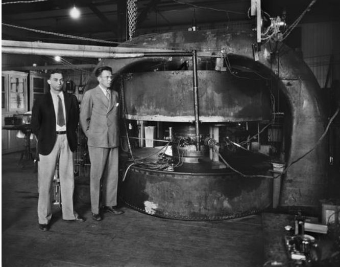
Livingston and Lawrence standing beside the 27 inch cyclotron, built in 1934
