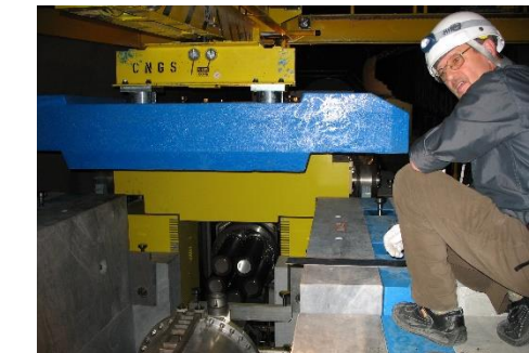
Installation of horn roof shielding
