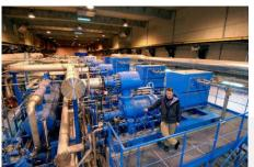
LHC Helium Refrigerators similar capacity required for P1 and for P5, in addition to 8 existing
