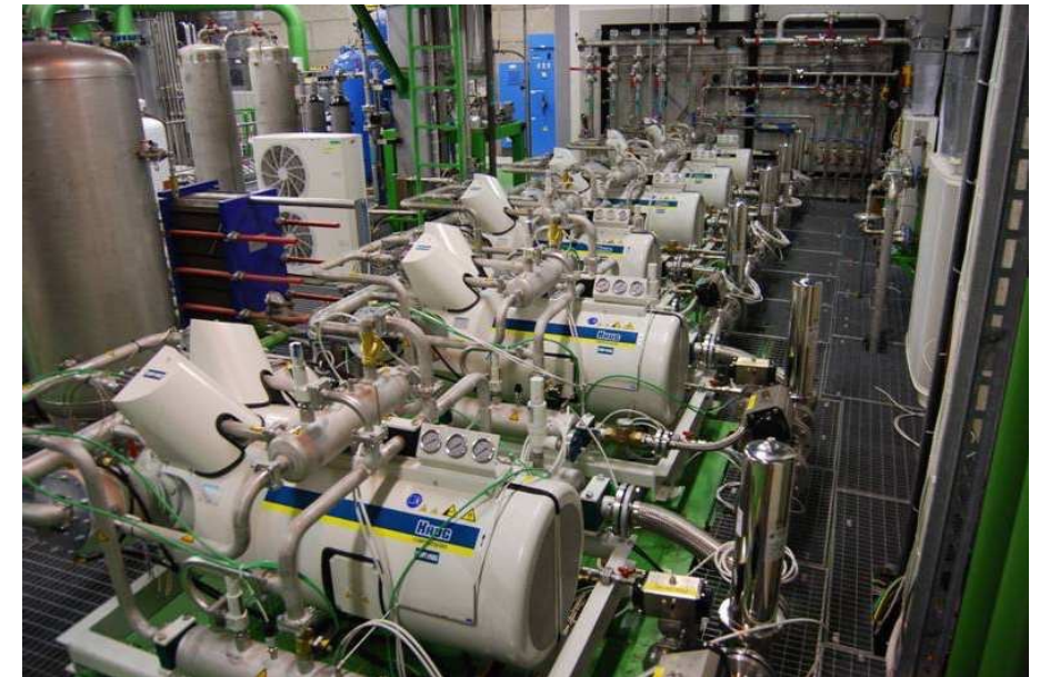
evaporative cooling system of ATLAS inner detector
