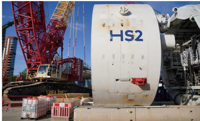
A tunnel boring machine at the HS2 site near Old Oak Common in west London. Photograph: Jonathan Brady/PA
