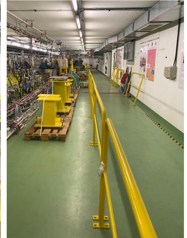
Equipment being evacuated
