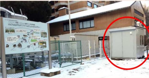
Panoramic view of the heat storage facility
