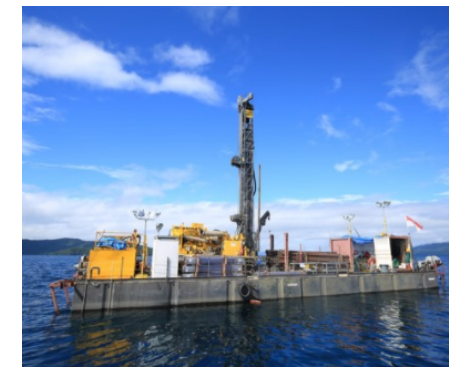
Drilling works on the lake
