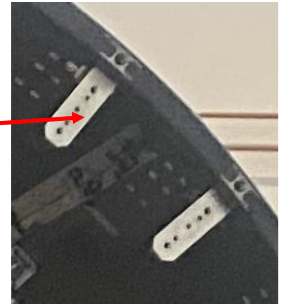
Angle Plates shown attached to inner skins by potted inserts
