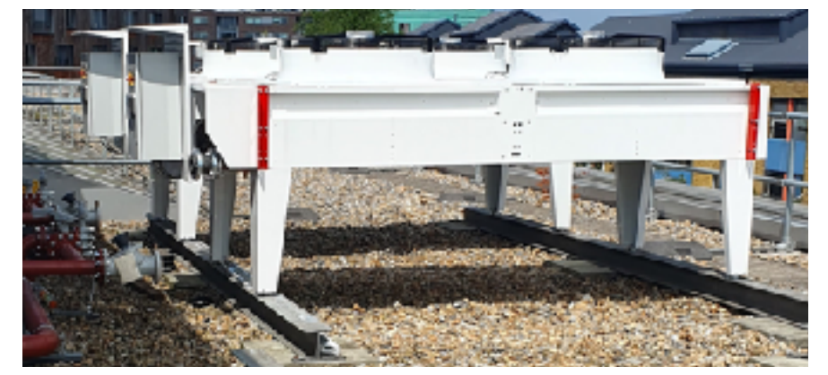
Dry air cooler 2 x 300 KW, PUE 1.3*
