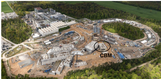
FAIR construction site, Apr. 2024
