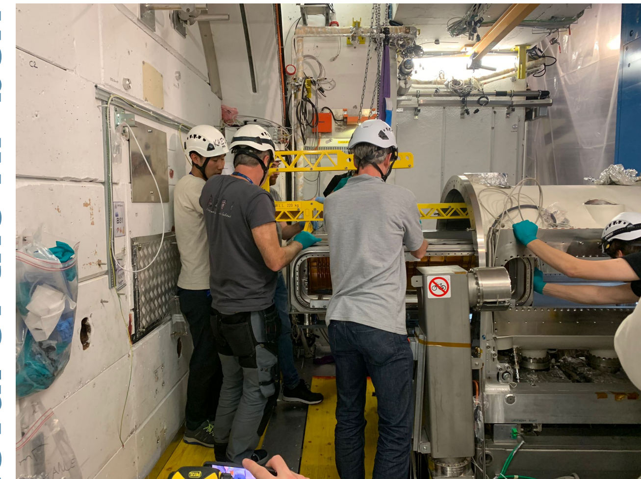
removal of the RF box
