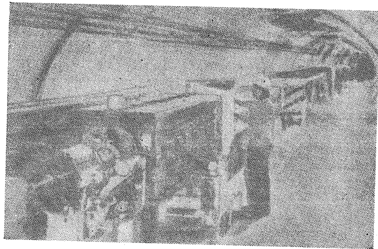
Fig. I.10. Inside SPS tunnel (Photo CERN)
