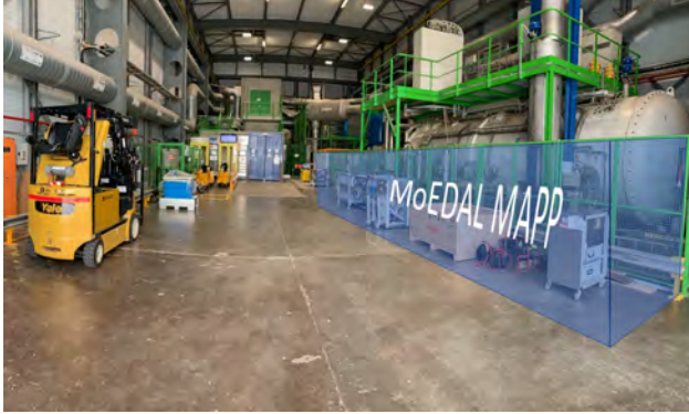
Fig. 19: The temporary staging area in SBD 2855.
