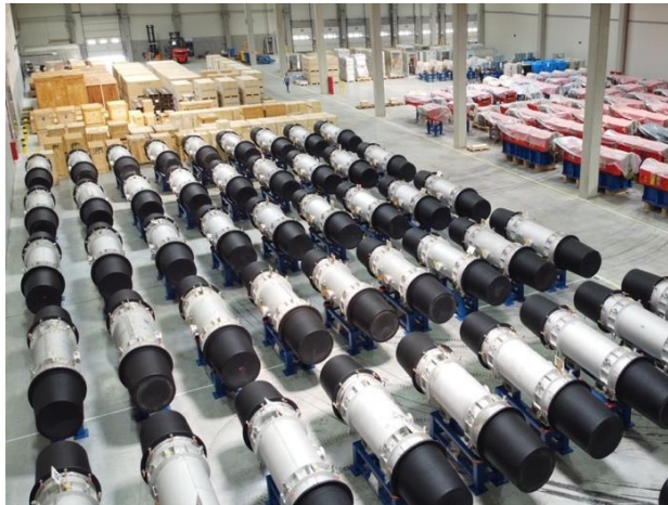
SIS100 dipoles ready for installation
