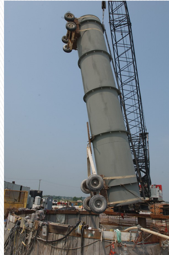
Large Equipment Rigging & Installation
