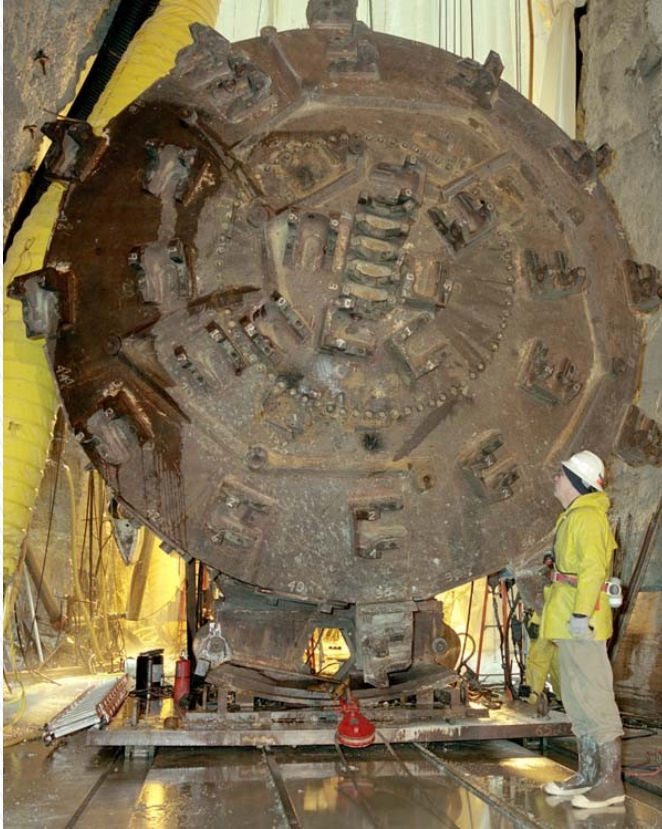
Tunnel Boring Machine
