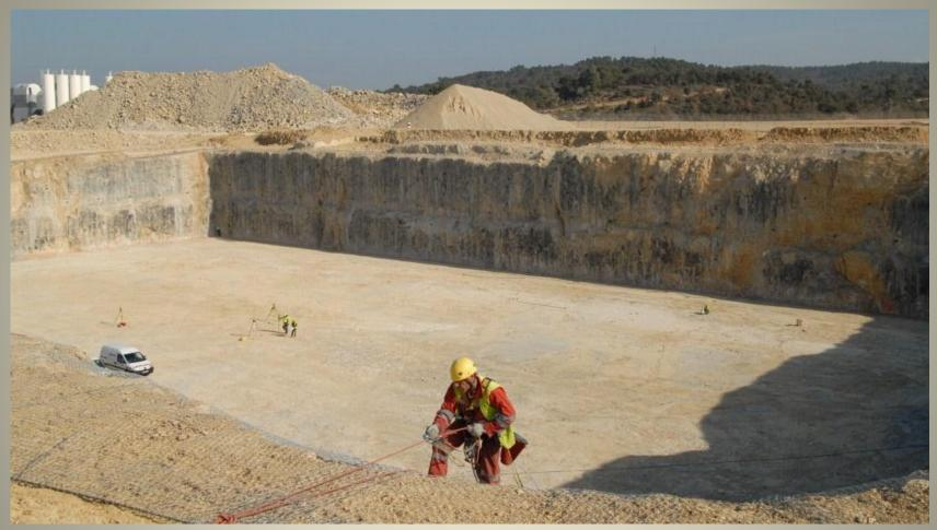
• March 2011 – the Tokamak pit – 17 m deep, 120 m long and 90 m wide - will house the anti-seismic foundations for the Tokamak Complex
