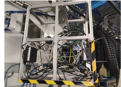
Complete installation with the buffering devices
