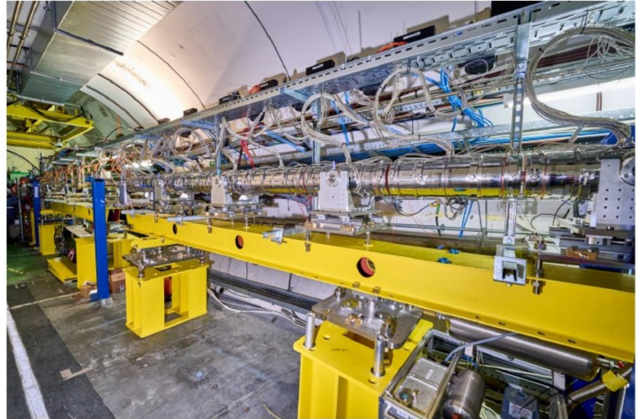
July 2023 – new vapour source installed
